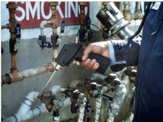
Test steam traps
